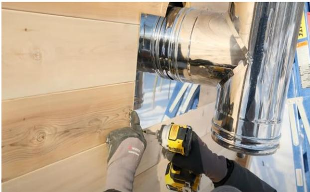
Install the bottom half of the exterior chimney shield using 1 ½" (38mm) screws ensuring it is level.
