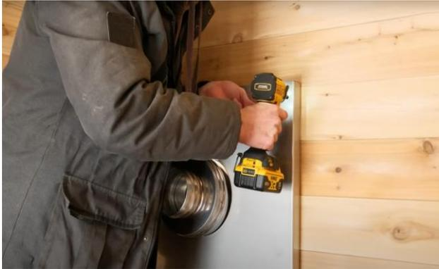
Center the heat shield around the hole and secure it to the wall with 6 - 1 ½" (38mm) screws in each of the holes.
