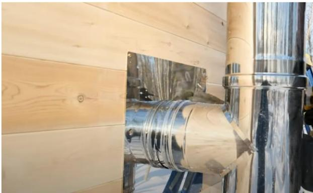
Overlap the top half of the exterior chimney shield and secure with provided screws.
