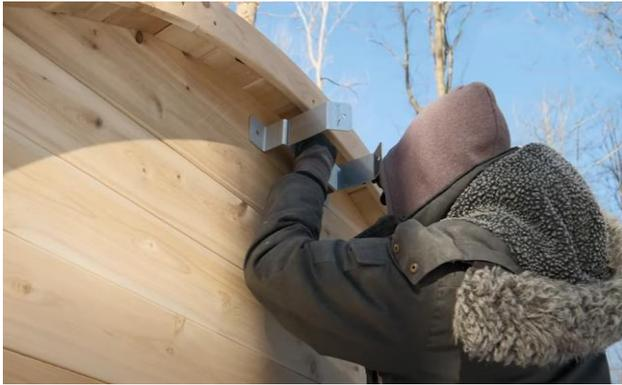
Place the assembled bracket onto the marks and secure to the wall with the provided lag screws.
