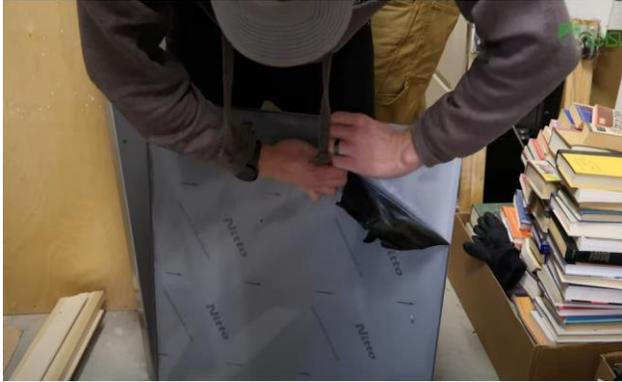
Before Starting the assembly of your TimberGlow wood heater, remove the protective film from the heater shield and floor plate.
