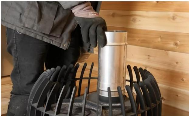
Place the shorter chimney connector piece onto the flange off the heater.
