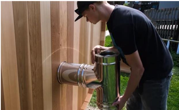
Insert the "T" chimney piece through hole from the back of the sauna through the rear wall heat shield on the inside of sauna and into the chimney connector.
