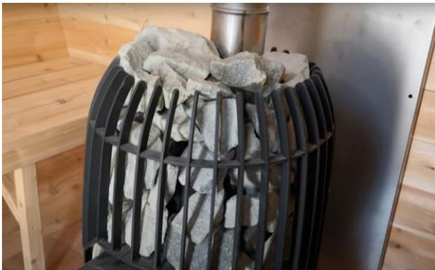
Place the rocks in the heater until they are 2" (51 mm) above the top of the heater.
