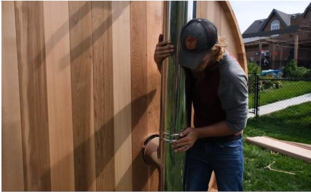
Attache assembled chimney pieces to the "T" coming out the back of the sauna and secure with the included bracket.
