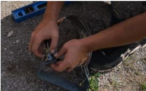
Remove the nuts and bolts from the chimney support.
