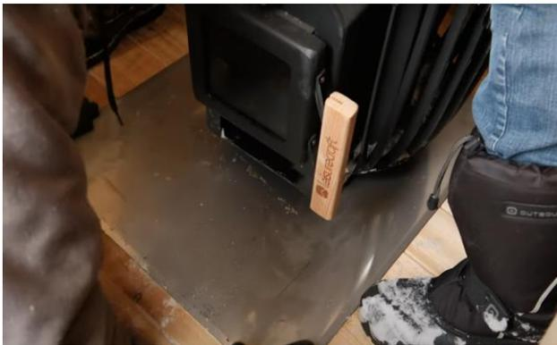
Place the stove in the correct position and center the floor plate under the stove.
