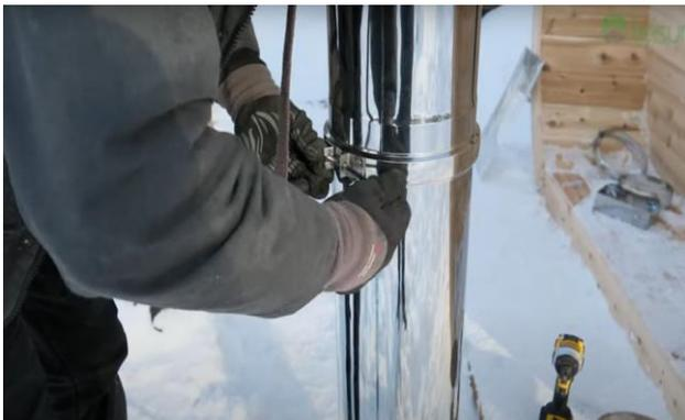
Remove the protective film from the chimney stacks.
