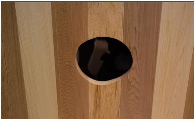
Cut out the opening with a jig saw.
