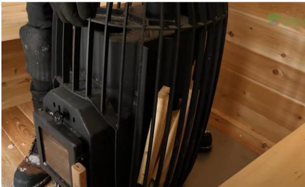
Bring the heater in and place it on top of the floor shield.
