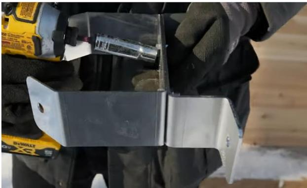
Secure the 2 wall brackets together with the provided nuts and bolts.
