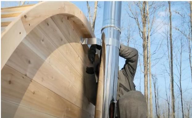
Attach the chimney to the bracket by placing the provided strap around the chimney and securing the strap to the bracket with the provided nuts, bolts, and washers.
