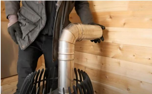
Connect the last chimney connector to the other end of the chimney.
