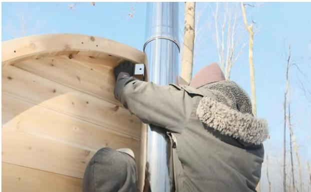
Place the wall support piece, ensure the chimney is level and mark the position of the sides of the wall support bracket.
