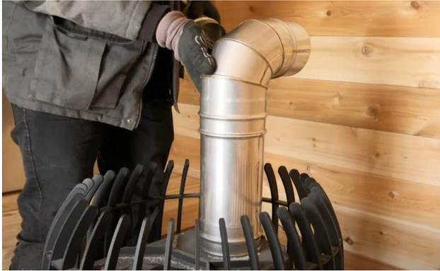
Connect the chimney elbow to the first chimney connector piece.
